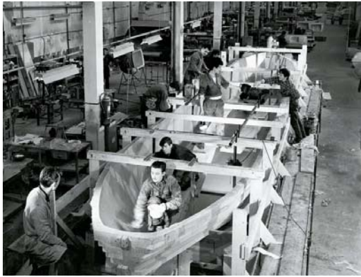
February 1967 – The Brittany model is well under construction: lots of manpower ...
